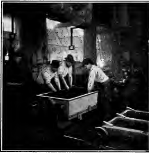
Fig. 59. Jolting the Drag Half of the Mould.
